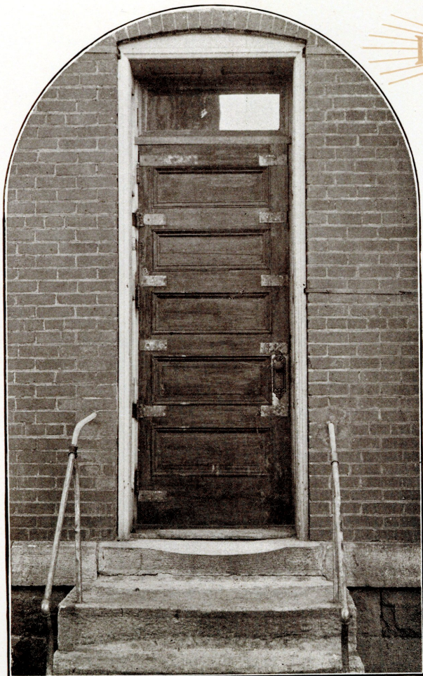
Old Door—Strong Portal
